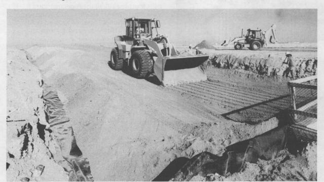
CAPPING IT OFF — A heavy equipment operator levels dirt during application of a final, topsoil layer of a demonstration landfill cover in Area 3. The work is being done as part of the Alternative Landfill Cover Demonstration project being conducted by Sandia for DOE.
